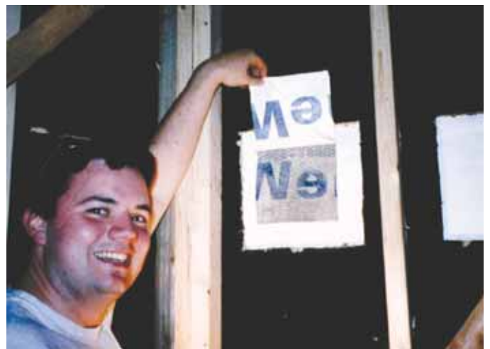
Photograph 6: Hardcoat Stucco Bonding to Plastic Building Paper —A young, happy engineer, discovers that stucco does indeed bond to plastic building papers preventing drainage. The engineer is my friend Chris Schumacher—may he remain this happy when he gets older.
